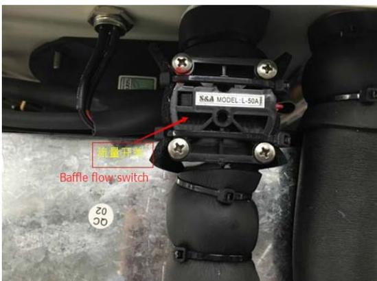
2) Cut off two red wires on the baffle flow switch, and then connect these two wires .Turn on the chiller to observe if the alarm continues.
