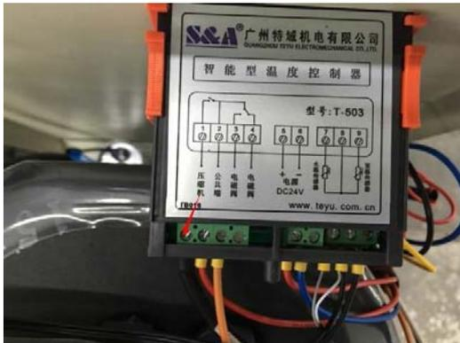
2.2) Check the working voltage output of output terminals of the solenoid valve at the back of thermostat with testing tools .If there is voltage output, it can be judged as thermostat failure, if no voltage output, then continue next testing.
