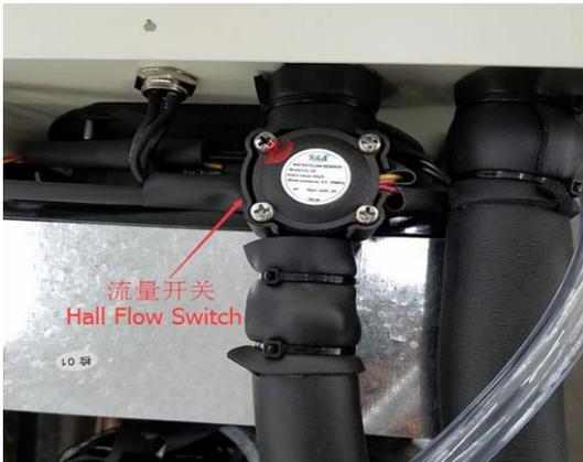
3) Cut off four wires on the Hall flow switch, connect the red wire with other red one, the black wire connect with the yellow one. And then turn on the chiller to observe if the alarm continues.
